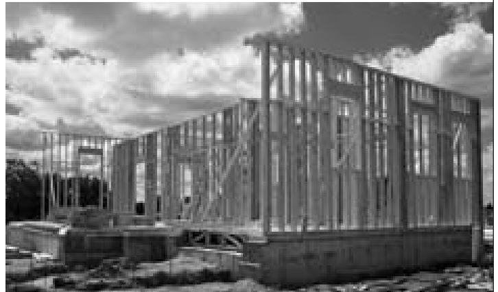
Automatic fire sprinklers help lower development costs, resulting in lower selling prices per unit.
