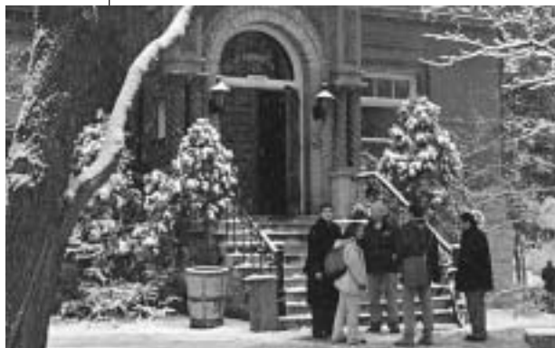
Over the next six years, Northwestern will retrofit 34 dormitories. In all, 65 buildings, including fraternities and sororities, will be retrofitted with fire sprinklers.
