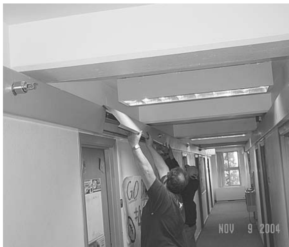
Sprinkler fitters (left) complete the project adding soffits and Burke Hall (right), the most recent residence hall, has been sprinklered.
